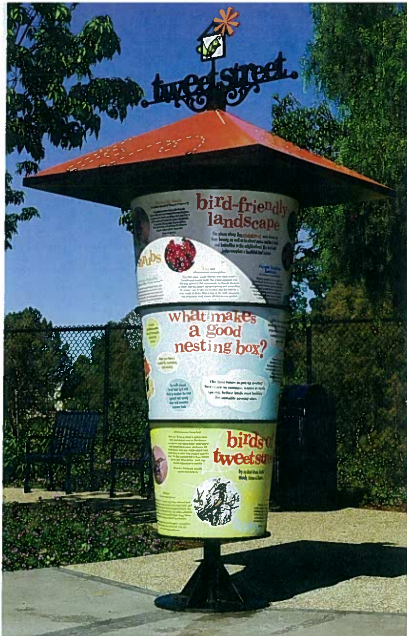
Above: The birdhouse-inspired interpretive kiosk features three conical aluminum panels, with graphics embedded in high-pressure laminate. Two of the three panels spin, but the third is stationary and embedded with Braille text.
